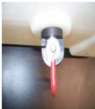
Fuel Valve ON:
